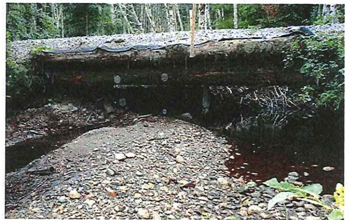
CK2263 From Downstream
